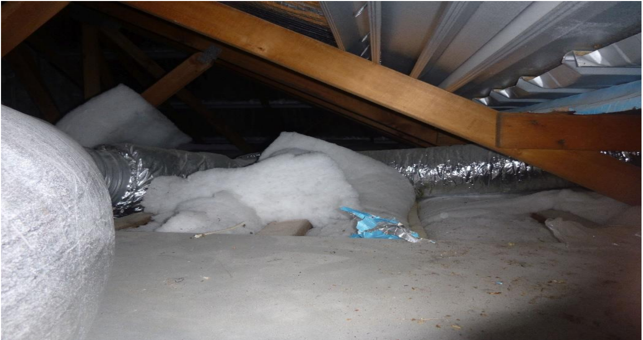
An example of insulation that has been disrupted and hence not providing the expected benefits
