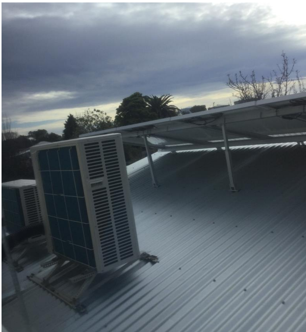
Solar panels and air conditioning units on the roof of a house
